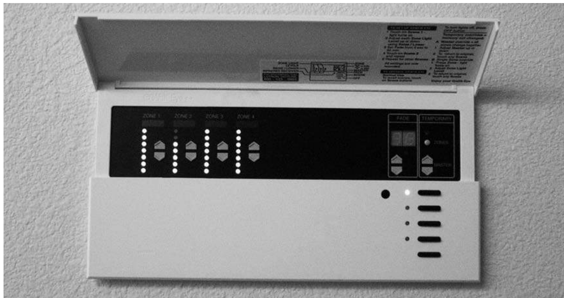
A Four Scene Four Channel Preset Dimmer (Lutron). Four Buttons Are Scenes—Four LED Ladders with Up Down Buttons Are the Four Channels, or Separately Dimmed Circuits
