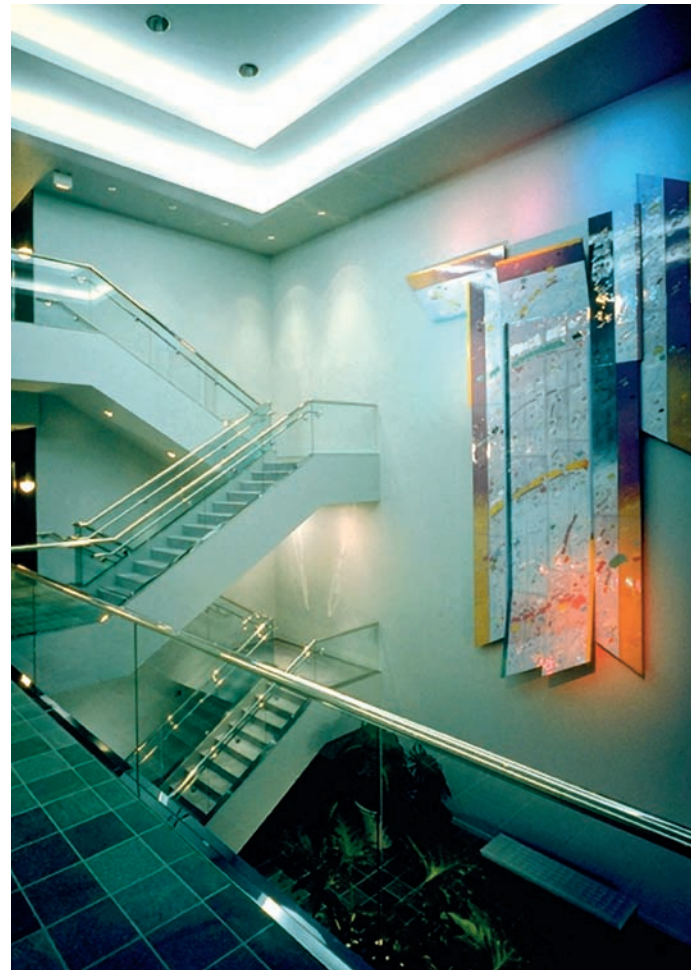
Plate 5-2 Building Lobby. Decorative lighting is limited to wall sconces by elevator doors (far left). Ambient light created by two step cove light. Task light created by downlight over stair and balcony. Focal light on wall art provided by concealed projector illuminators using color filters. Photo: J. Benya
